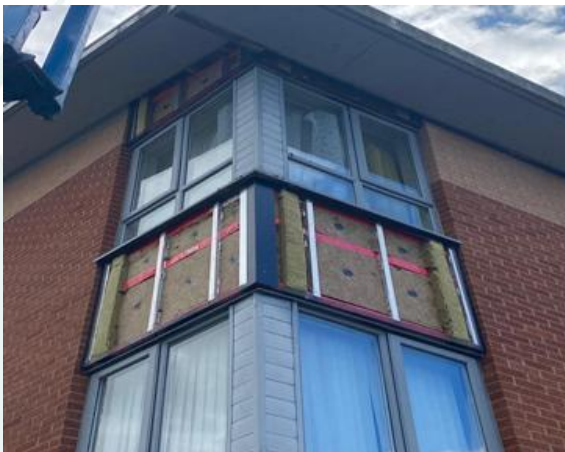
D/E – Now Ready For Panels
