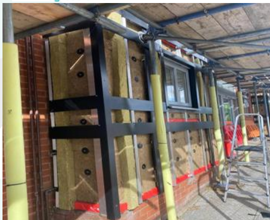
B1 Now Ready For Fire Stop & Insulation
