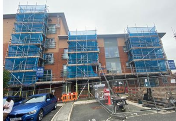
A Photo Showing That We Are Now Ready For Panels
